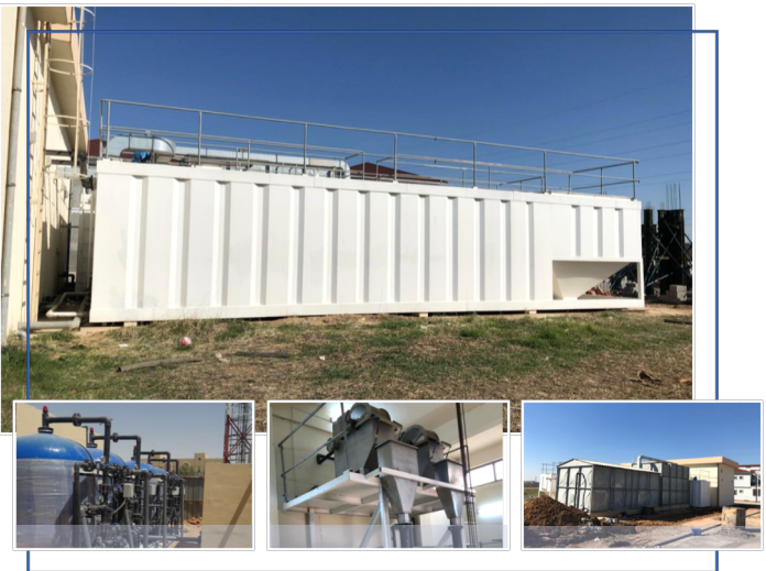
Qaiwan Heights 1,000 m3/day MBBR wastewater treatment plant in slemani
