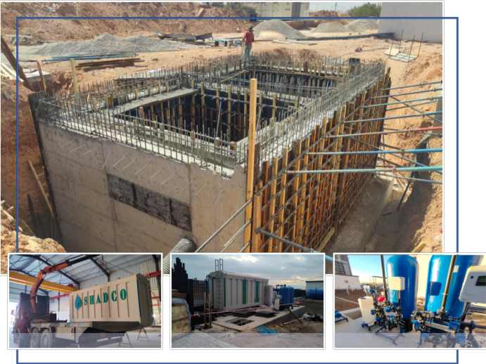
Khawnakan Complex 100 m3/day MBBR underground wast water in slemani
