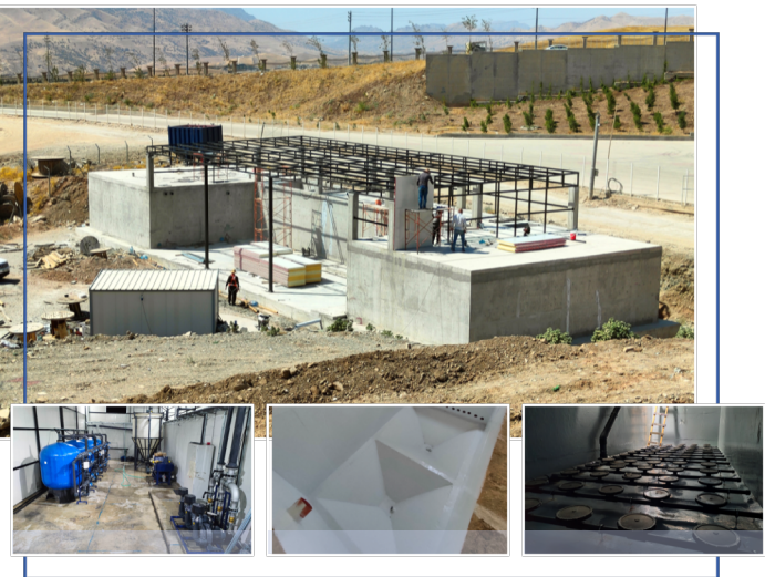
Khawnakan Complex 100 m3/day MBBR underground wast water in slemani
