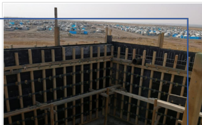
TEARFUND organization: construction 300m3 water tank in salameya :2020
