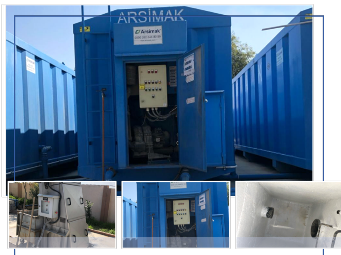
400 m3/day MBBR wastewater treatment plant, located oil company
