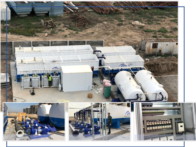
Slemani Heihgts 1,000 M3/day MBBR wastewater treatment plant in slemani
