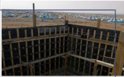
TEARFUND organization: construction 300m3 water tank in salameya :2020
